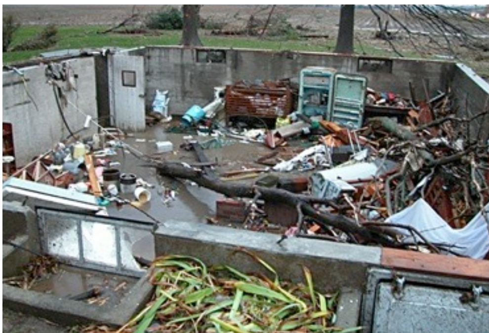
This debris-strewn basement is all that remains of rural Van Wert resident Mary Germann's home after an F-4 tornado went through the county on November 10, 2002. Dave Mosier/ Van Wert independent
